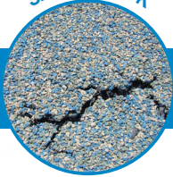
SPIDER CRACK
